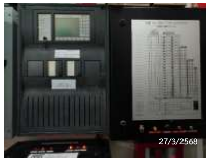
Fire Alarm Control Panel
